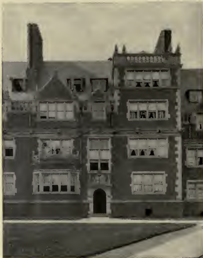
DETAIL OF DORMITORIES
