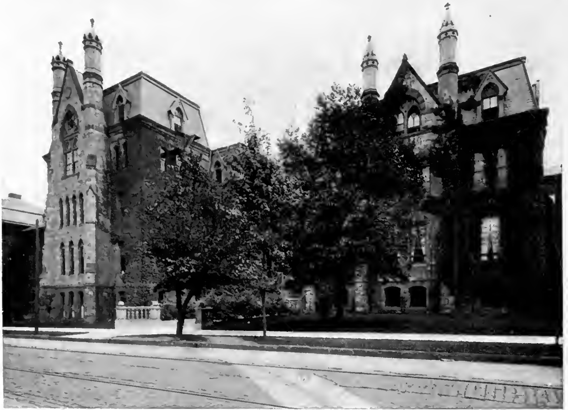
MAIN HOSPITAL BUILDINGS
