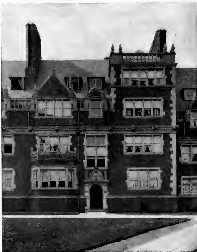
DETAIL OF DORMITORIES
