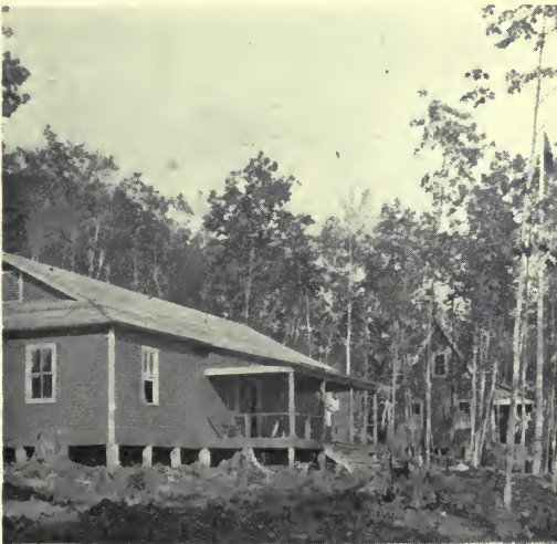
MAIN BUILDING AND STAFF OFFICES
