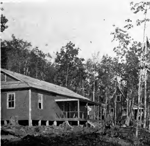
MAIN BUILDING AND STAFF OFFICES
