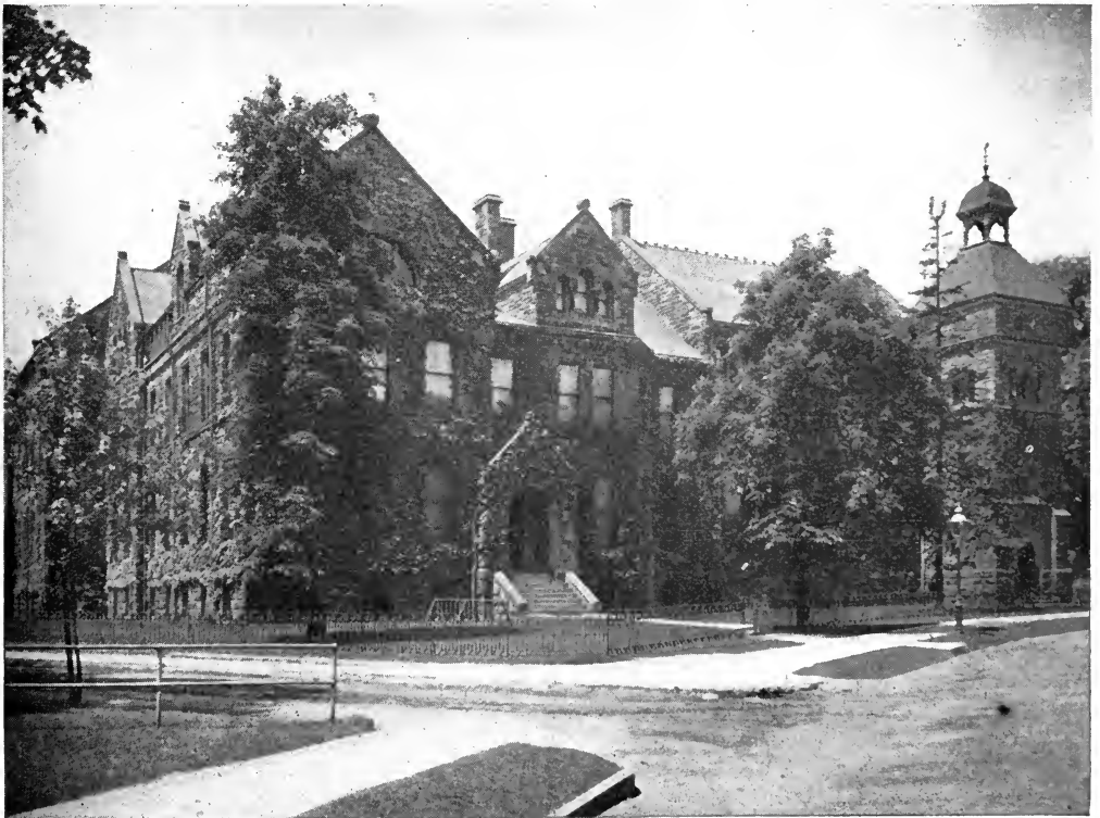
BIOLOGICAL BUILDING, from Queen's Park The new Anatomy Building is to be erected on the right
