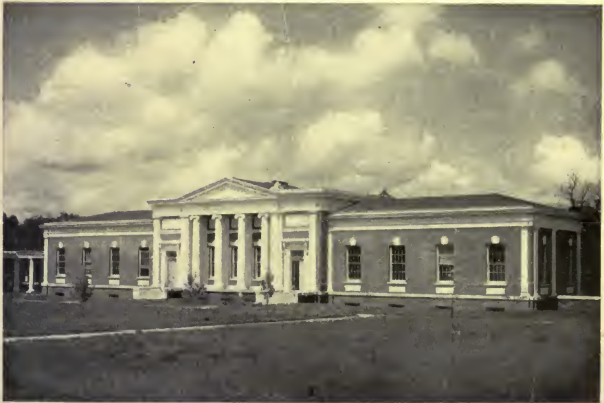
University—Mechanical Laboratory (Erected 1896-98)
