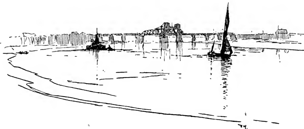
KING'S FERRY BRIDGE.
