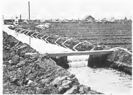
Farm irrigation system, showing distribution ditch, well pump (upper left), check gate for controlling flow in the ditch, and siphons to carry the water from ditch to furrows
