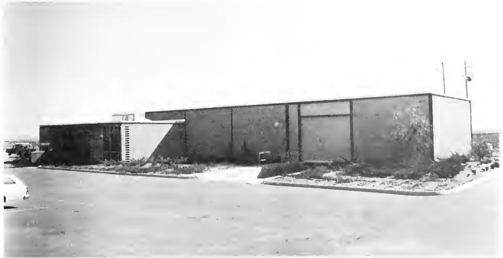
Structure typical of many Department of Water Resources' buildings that are being modified for passive energy conservation
