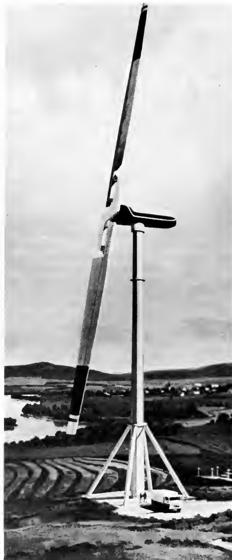
Artist's rendering of an experimental wind turbine to be built to develop wind energy systems and test their potential for producing energy. It is designed for use at sites where the average wind speed is 22.4 kilometres per hour. The 90-metre-long rotor is supported on a 60-metre high tower. The generator will produce 2 500 kilowatts of electricity. Called "the largest windmill in history," the wind turbine is to be built by Boeing Engineering and Construction Company under an Energy Research and Development Administration program managed by the National Aeronautics and Space Administration. Courtesy Boeing Engineering and Construction Co.
