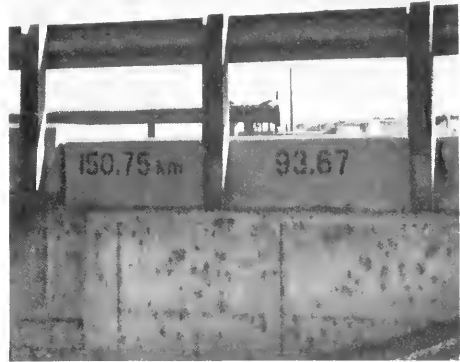
Bridge in Fresno County across the California Aqueduct displays both mile-point and kilometre markings
