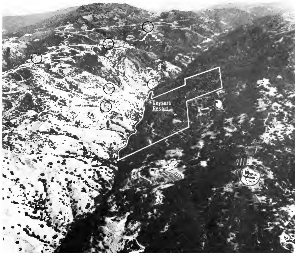
Future site of DWR's South Geysers Powerplant in the Mayacmas Mountains in Sonoma County, an area of abundant geothermal activity. This facility, which is planned to generate 55 000 kilowatts,
