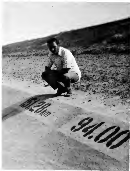
One of the mile point markers (94.00) originally used along the California Aqueduct is supplemented by its metric equivalent in kilometres.
