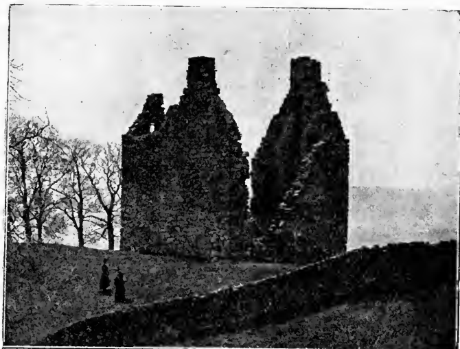
Frenchland Tower, remains of old Ash Avenue.
