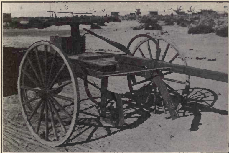
FIG. 23.—Twin Falls sage brush grubber.
