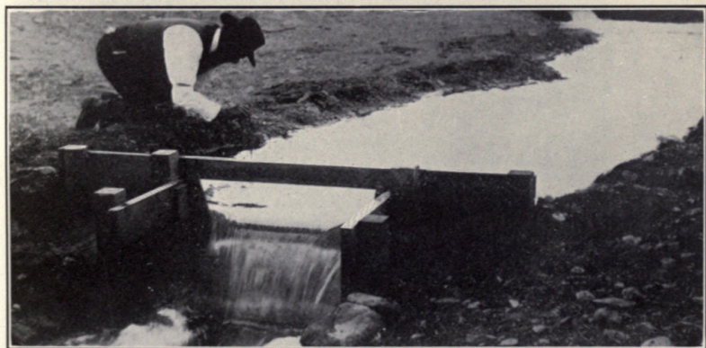
FIG. B.—Upstream view showing measurement being taken.
