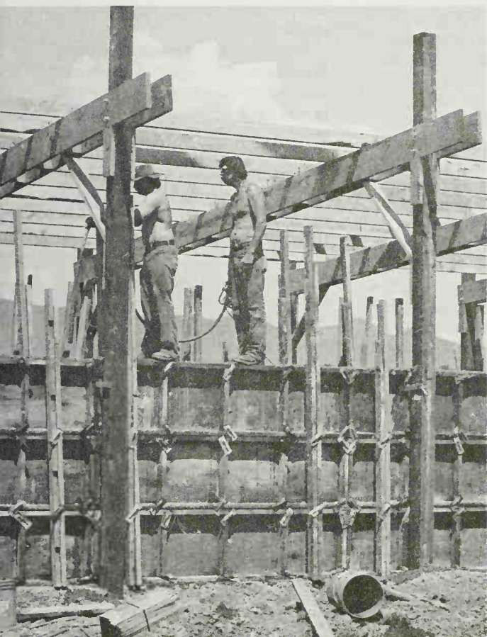
Construction jobs were yet another benefit of the Rural Clean Water Program in Tillamook County. Here, carpenters build a dry manure storage structure that will have a roof to deflect the high annual rainfall in the area.
