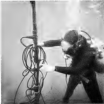
The diver connects phone plug into any station located throughout the underwater portion of the tower arrays.
