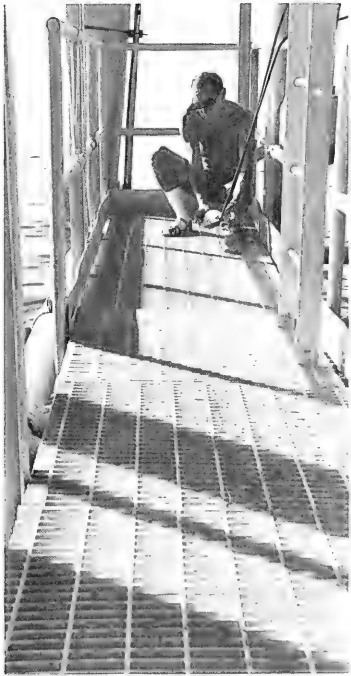
Long landing, loading, and working platform near the water surface extends along the east side. Surface collections and measurements are made from this steel grating catwalk.
