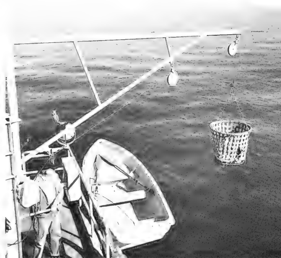
Supplies and equipment are transferred from boat to tower by means of a 700-pound capacity nylon basket attached to this 18-foot loading boom. Combination workboat and lifeboat stands ready for use (left, foreground). It is lowered with the same boom.
