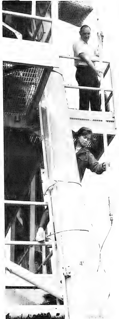
Installing tide gauge.
