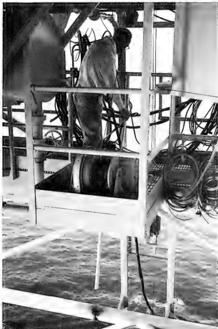
Technician operates winch controlling west rail cart while paying out signal and power cable. Exchangeable cables and hoses are attached to the hand rail on this deck.
