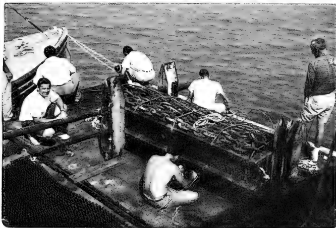
Figure 3-9b. Inner Mooring Coral Hook on Deck of Pontoon Barge
