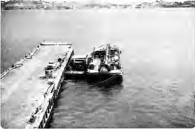
Figure 5-3a. YC-1378 Outboard of Pontoon Barge Loading Cable under Tension
