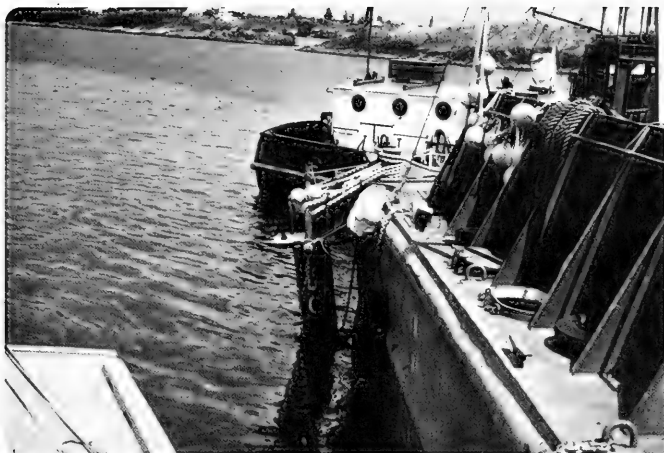
Figure 3-9a. Outer Mooring Coral Hook Slung Over Side of Cable Laying Barge
