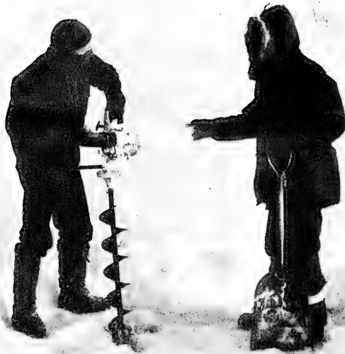
Figure 5.b. Drilling Instrument-Access Hole
