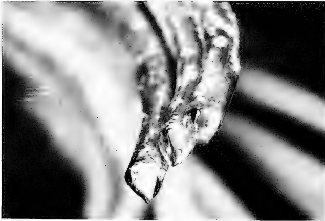
Figure 4-2. Bitter End of Signal Cable Slipped out of Termination 1B
