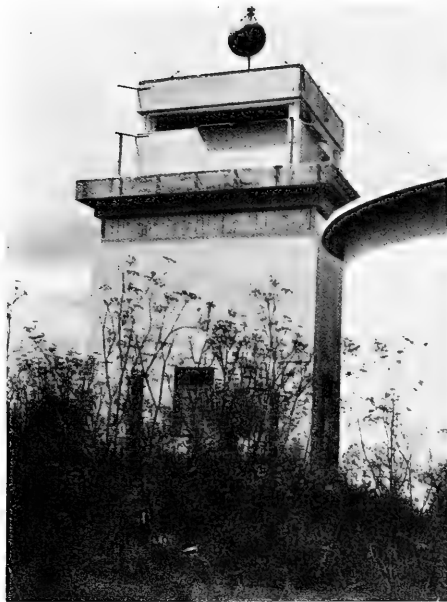
Figure 5-2a. Paynters Hill Tracking station
