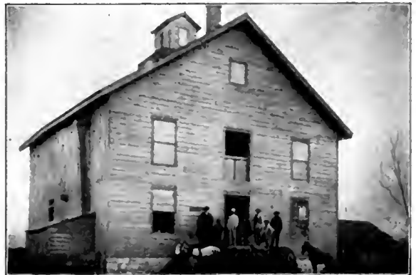
EXCELSIOR ROLLER FLOUR MILLS.
