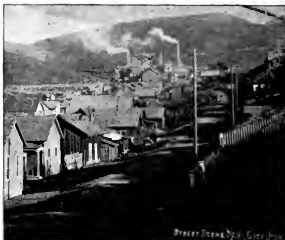
PARK CITY STREET SCENE, SHOWING ONTARIO MILLS.
