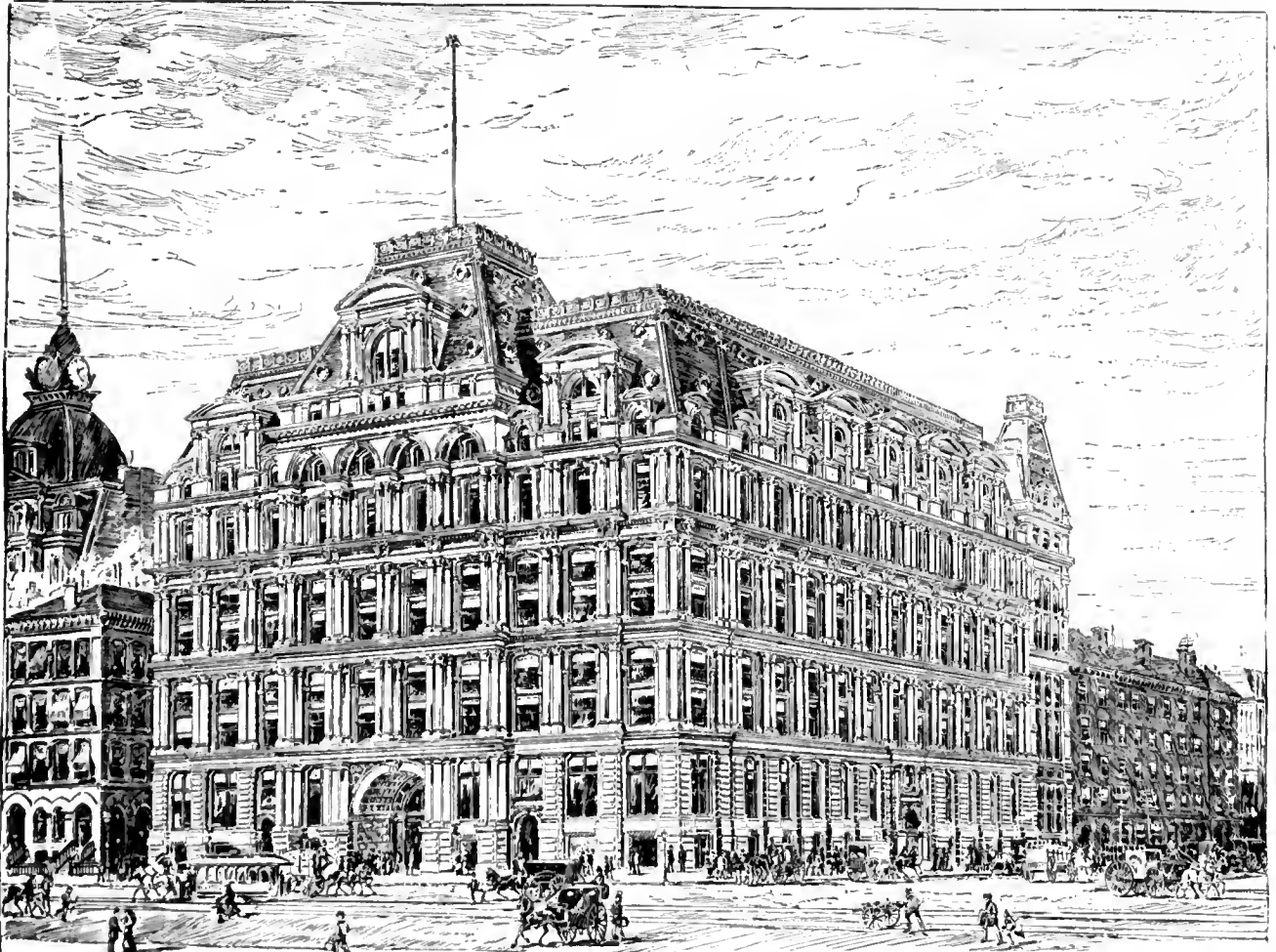
EQUITABLE LIFE ASSURANCE BUILDING, NEW YORK.
