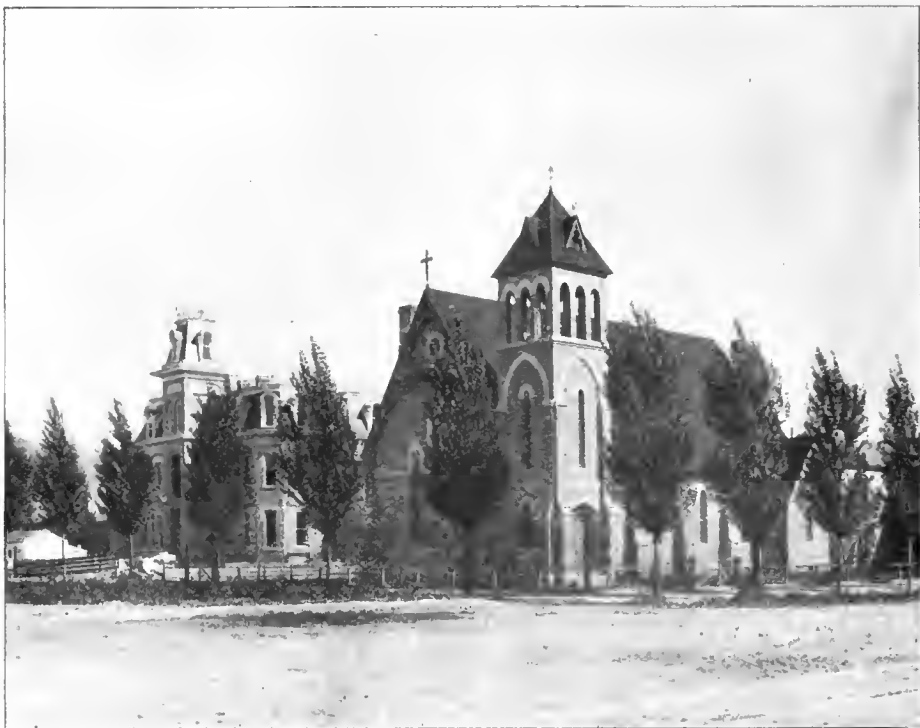
ST. MARK'S CATHEDRAL (EPISCOPAL) TWO AND A HALF BLOCKS EAST OF MAIN STREET, NORTH SIDE OF FIRST SOUTH.
