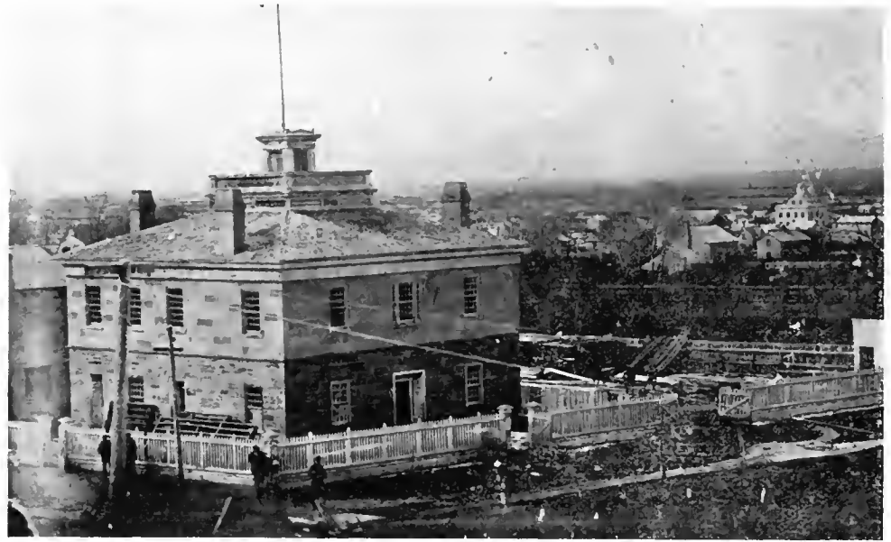
THE OLD COUNCIL HOUSE, WHERE THE FIRST COURTS WERE HELD IN UTAH.
