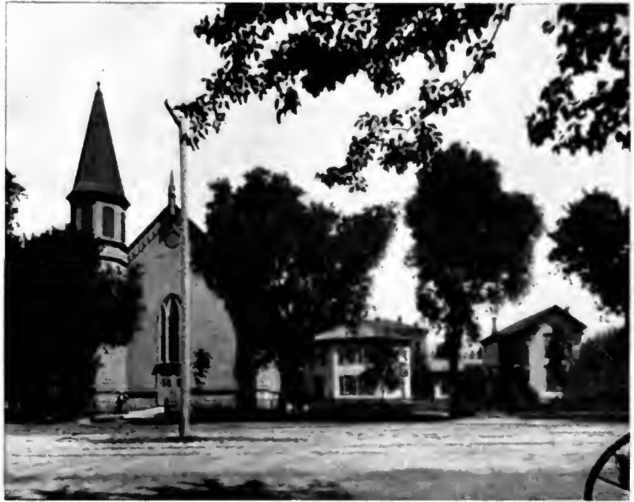
PRESBYTERIAN CHURCH, CORNER HASSING SOUTH AND HASSING EAST STREETS.
