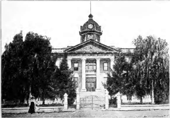
BOXELDER COUNTY COURTHOUSE, BRIGHAM
