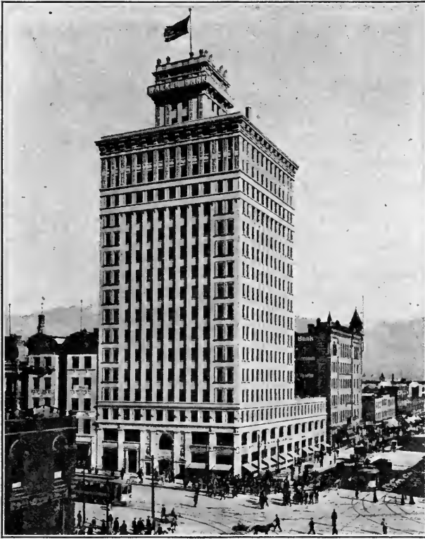
WALKER BANK BUILDING, SALT LAKE CITY
