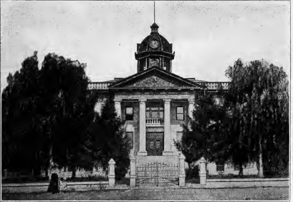
BOXELDER COUNTY COURTHOUSE, BRIGHAM
