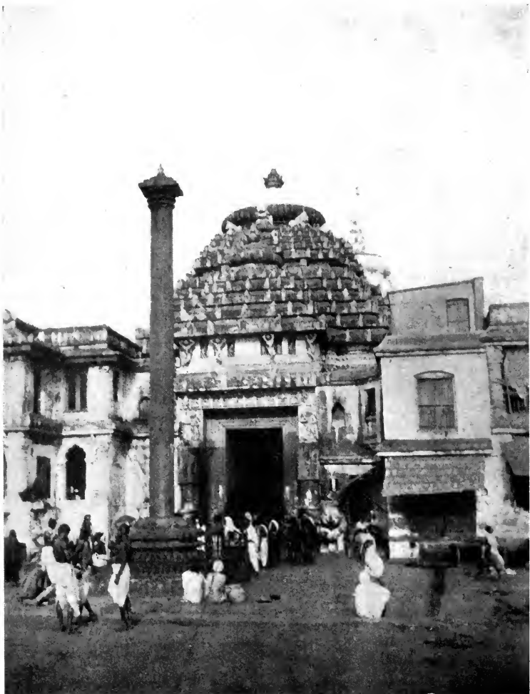
The main entrance to Juggernaut's temple in Puri. I was mobbed for stepping on the flagging around the column
