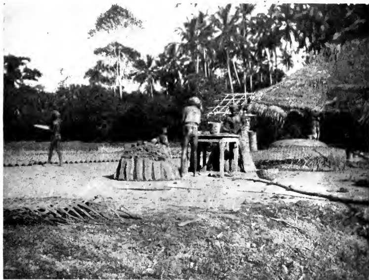
Central Ceylon. Making roof-tiles. The sun is the only kiln
