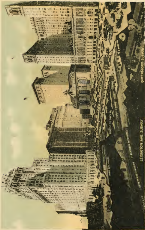
THE BOWMAN GROUP, SHOWING THE COMMODORE, BILTMORE, BELMONT AND THE PROPOSED NEW MURRAY HILL, AT GRAND CENTRAL TERMINAL
