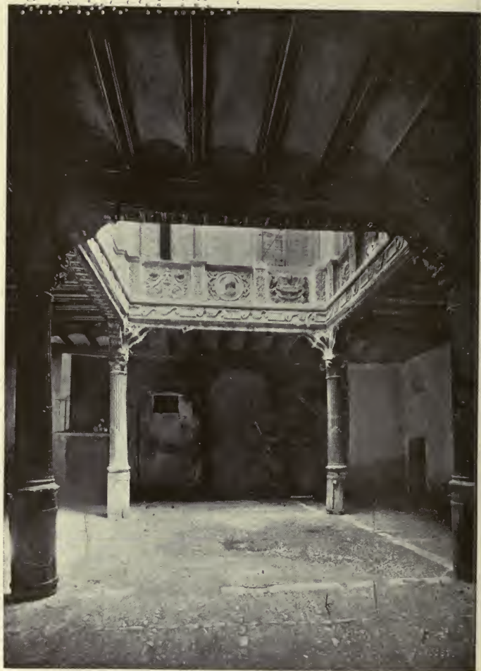
COURT-YARD IN THE HOUSE OF PARDO. ZARAGOZA
