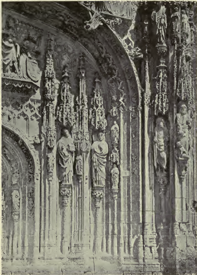
DETAIL OF THE RIGHT-HAND SIDE OF THE PORCH OF ST. PABLO VALLADOLID
