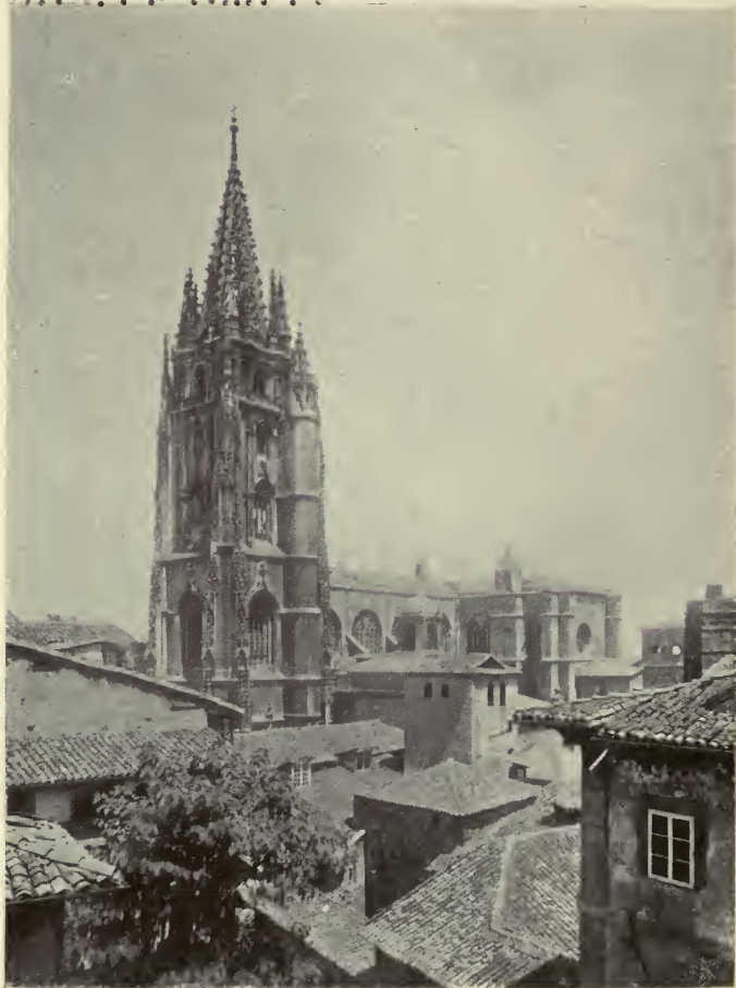
TOWER OF THE CATHEDRAL OVIEDO
