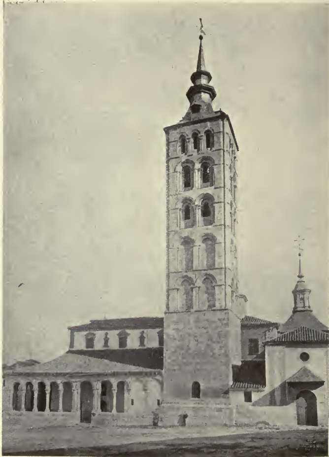
GENERAL VIEW OF ST. STEPHEN SEGOVIA
