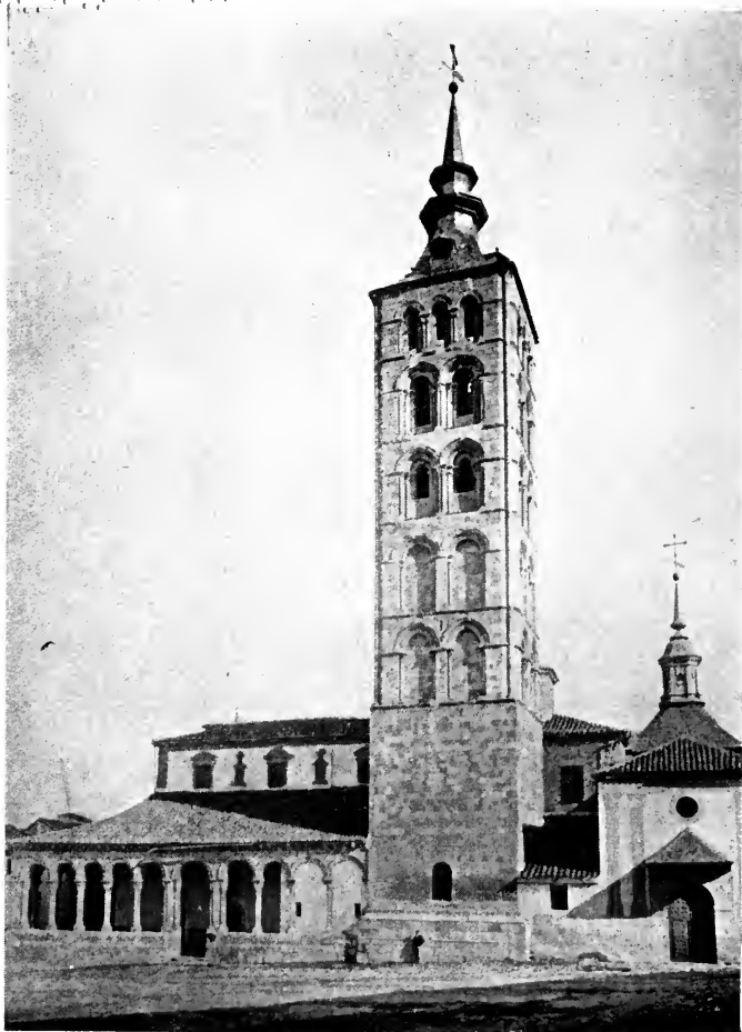
GENERAL VIEW OF ST. STEPHEN SEGOVIA
