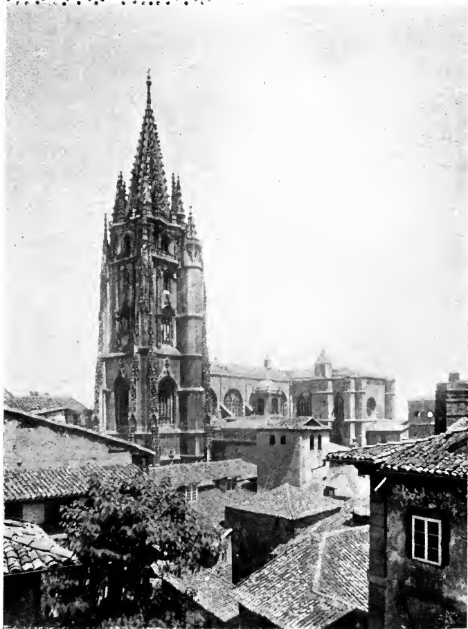
TOWER OF THE CATHEDRAL OVIEDO
