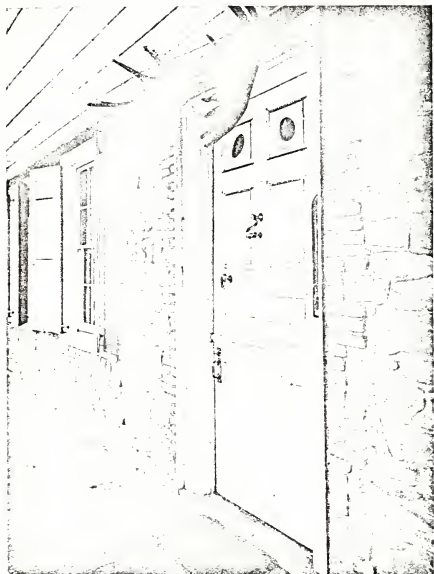
THE FRONT DOOR OF THE MANOR HOUSE, SHOWING LOOP HOLES FOR DEFENCE
