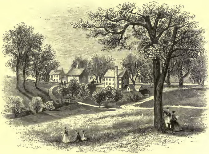
THE PUMP-HOUSE AND ITS SURROUNDINGS.
