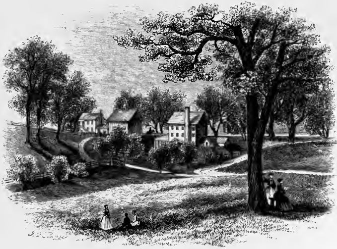
THE PUMP-HOUSE AND ITS SURROUNDINGS.
