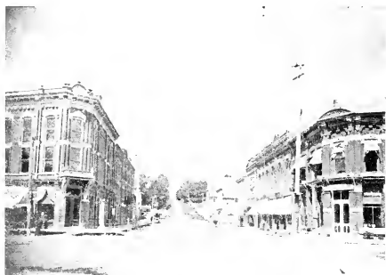
HURON AVENUE--Looking West
