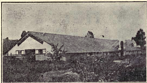
FIG. 80. CELERY STORAGE HOUSE
