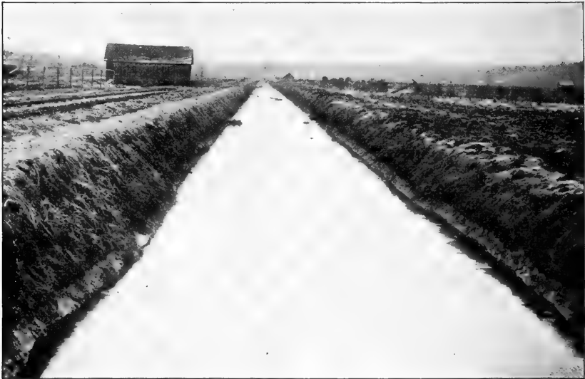
FIG. 450.—SLATE DITCH AT SOUTH LIMA, N. Y. CELERY LAND ON EITHER SIDE
