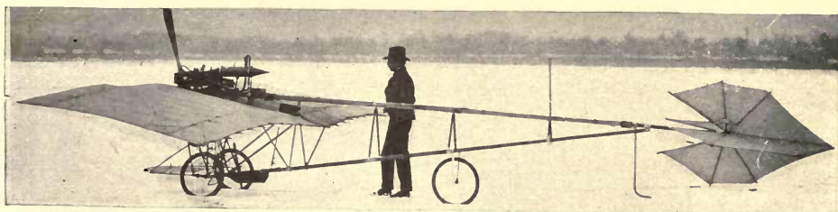
FIGURE 219.—Side View of Santos-Dumont's "Demoiselle."
