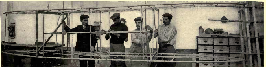
FIGURE 196.—Elevator Frame of Wright Machine.
