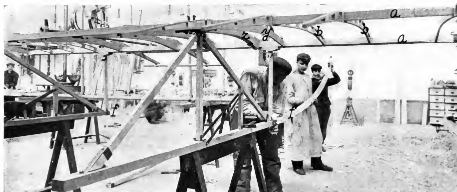
FIGURE 193.—The Wright Runner Construction. The solid ribs yz serve to support the motor, operator, etc. The other ribs bb are so built up as to enclose the wing bars aa between the double surfacing of fabric. The attachment of the forward curved members of the runners at f is clearly apparent upon close examination.
