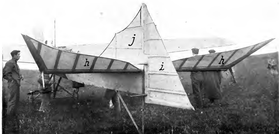
FIGURE 85.—Rear Controls of Antoinette Monoplane. In this hh are horizontally-pivoted surfaces for steering up or down; i is a vertically pivoted surface for steering sidewise; and j is a vertical fin used for its stabilizing effect.
