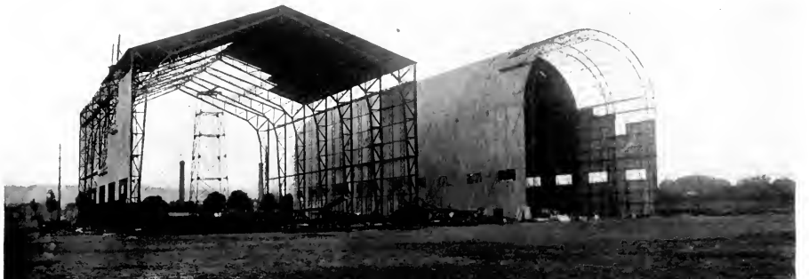
FIGURE 16.—Balloon Houses Nearing Completion.
