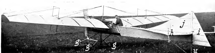
FIGURE 216.—Rear View of Antoinette VII. This is the machine with which Latham flew 20 miles in his second attempt to cross the English Channel. Ailerons are discarded in favor of rocking the whole wing, and the alighting gear is reduced to the wheels g g g and u .
