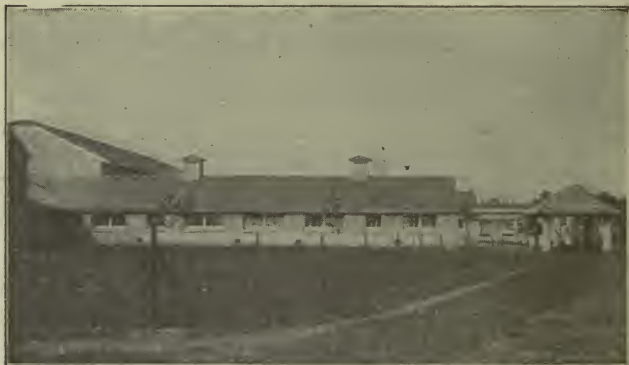
Fig. 25.—Low ventilating flues having their efficiency much reduced by closely louvred shelters, diminishing the effect of the wind in producing draft.
