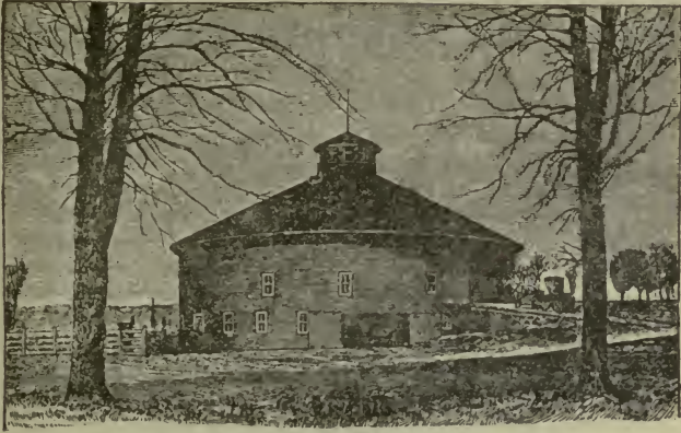
Fig. 51.—First barn in which the King system of ventilation was installed, in 1889.
