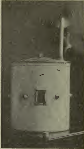
Fig. 15.—Wind across ventilator increases draft.
