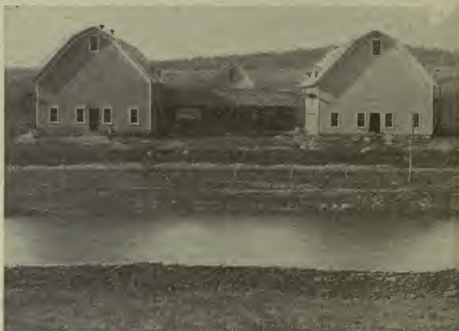
Fig. 23.—Showing improper installation of ventilating flues just above the eaves. In such cases whenever the wind is from the opposite direction the tendency will be to give a much reduced draft or even reverse its direction, causing it to be downward into the stable.
