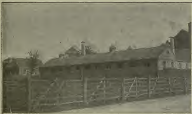
Fig. 26.—Ventilating flues rising high above the roof and with outlet sheltered so as to permit free wind movement and easy escape of air from the flues.
