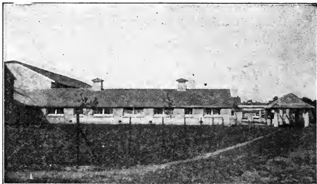
Fig. 25.—Low ventilating flues having their efficiency much reduced by closely louvered shelters, diminishing the effect of the wind in producing draft.
