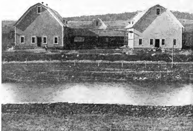
Fig. 23.—Showing improper installation of ventilating flues just above the eaves. In such cases whenever the wind is from the opposite direction the tendency will be to give a much reduced draft or even reverse its direction, causing it to be downward into the stable.
