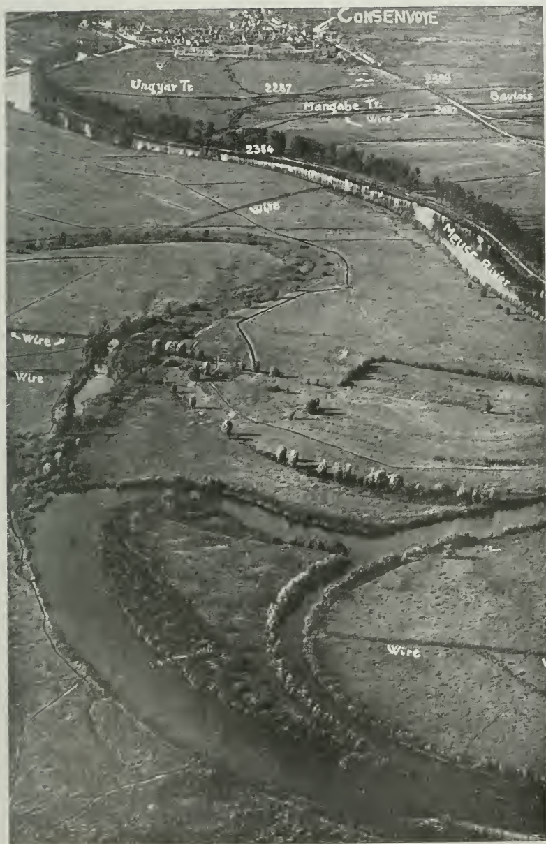
THE VALLEY OF THE MEUSE TO THE SOUTH OF CONSENSVOYE. A French protograph used in the preparation of the American offensive on the banks of the Meuse in September 1918. The barbed-wire entanglements and trenches are plainly indicated.
