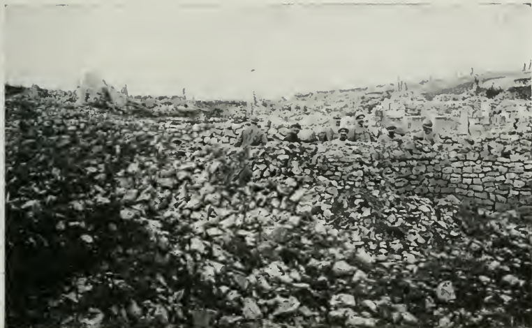
A TRENCH IN THE RUINS OF AVOCOURT IN APRIL, 1917.
