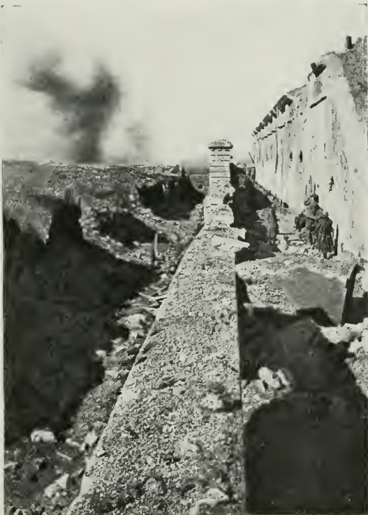
THE SOUTH MOAT OF VAUX FORT IN MAY 1916.
