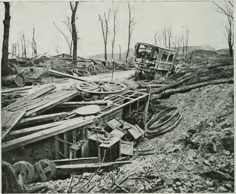
THE ROUTE DU FORT TAVANNES IN JUNE 1916.
