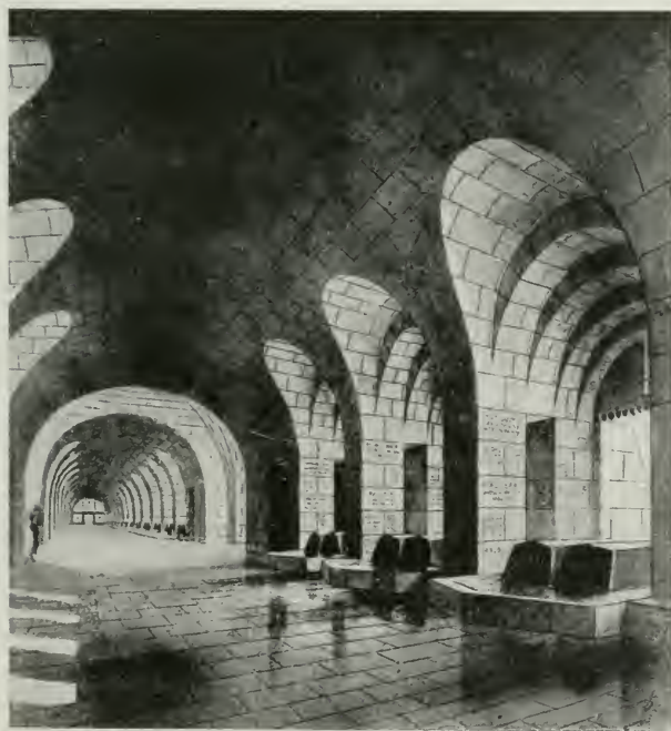
CLOISTER OF THE MORTUARY OF DOUAUMONT.— RECESSES FOR THE TOMBS.
