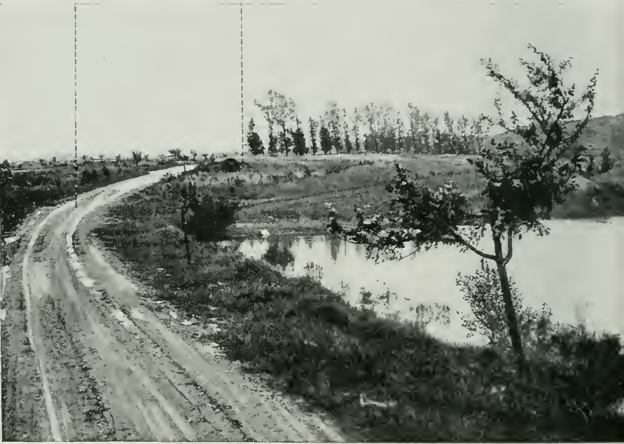
PANORAMIC VIEW OF VAUQUOIS CREST TAKEN
