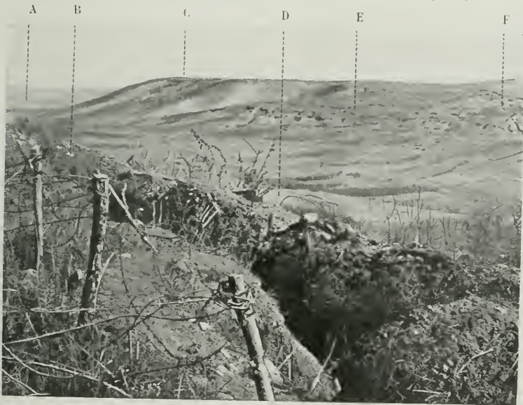
GENERAL VIEW OF THE EPARGES RANGE, TAKEN FROM THE CREST OF MONTGIRMONT A. The Woëvre. — B. The trench from which the photo was taken, on the crest of Montgirmont. — C. The Eparges crest. — D. Mort ravine. — E. Dug-outs on the side of Eparges Hill, F. A Trench.
