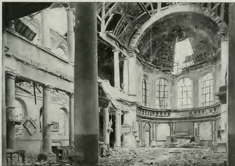
THE INTERIOR OF THE CHURCH OF SAINT-SAUVEUR IN AUGUST 1916.
