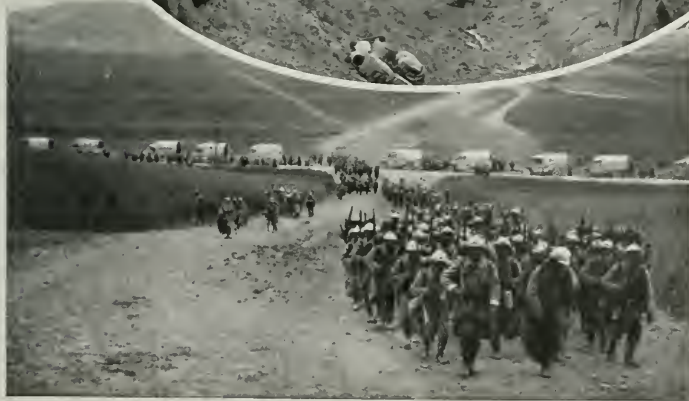
RE-INFORCEMENTS ARRIVING ON THE "SACRED WAY" (MARCH 1916).
