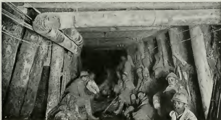
CORBEAUX TUNNEL AFTER ITS CAPTURE (AUGUST 22ND 1917).
