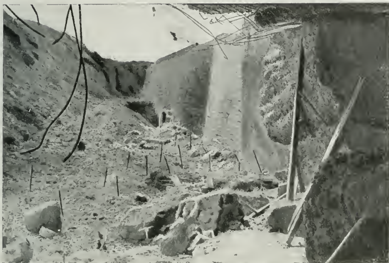
THE NORTH-EAST MOAT OF VAUX FORT IN APRIL 1916. View of the north casemate demolished by the bombardment.
