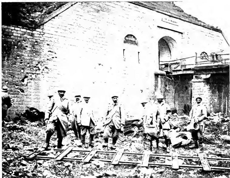
THE SOUTHERN MOAT AND ENTRANCE TO TAVANNES FORT IN JUNE 1916.
