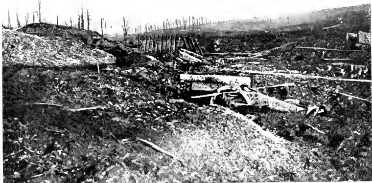
FONTAINES RAVINE IN FEBRUARY 1917. — A demolished French battery.
