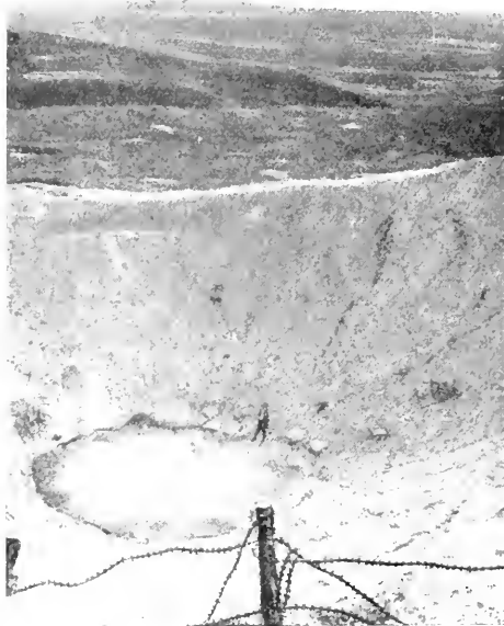
A MINE CRATER AT THE EXTREMITY OF THE SPUR, POINT X. (60 METRES IN DIAMETER, 30 IN DEPTH).
