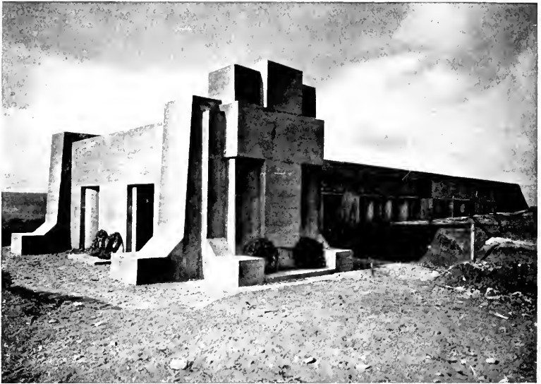
THE MONUMENT OF "BAYONET TRENCH" (A. Ventre, architect). On the right, the trench leading to the porch of the monument.
