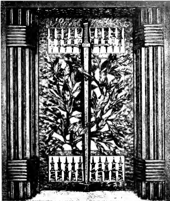
THE WROUGHT IRON GATE OF THE ENTRANCE PORCH OF THE MONUMENT, carried out by M. E. Brandt, art iron-worker (101, Boulev. Murat, Paris).
