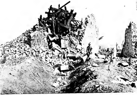
BRAS CHURCH WITH THE RUINS OF THE STEEPLE (APRIL 1917).
