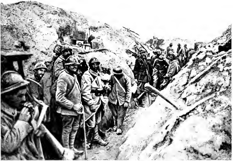
MORT-HOMME. — IN THE CAPTURED TRENCHES (AUGUST 1917).
