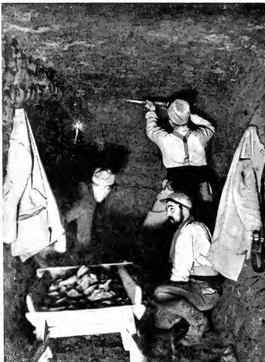
SAPPERS EXCA- VATING A MINE GALLERY.
