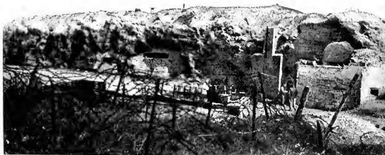
VAUX FORT. — THE CASEMATES OF THE GORGE OF THE FORT. The moat has been filled up by the bombardment.
