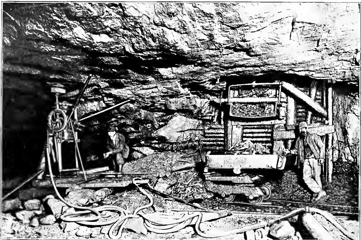
B. FILLING SYSTEM, MINNESOTA MINES, SOUDAN, MINN., WITH CHUTE FOR DISCHARGING REFUSE FROM UPPER LEVELS.
