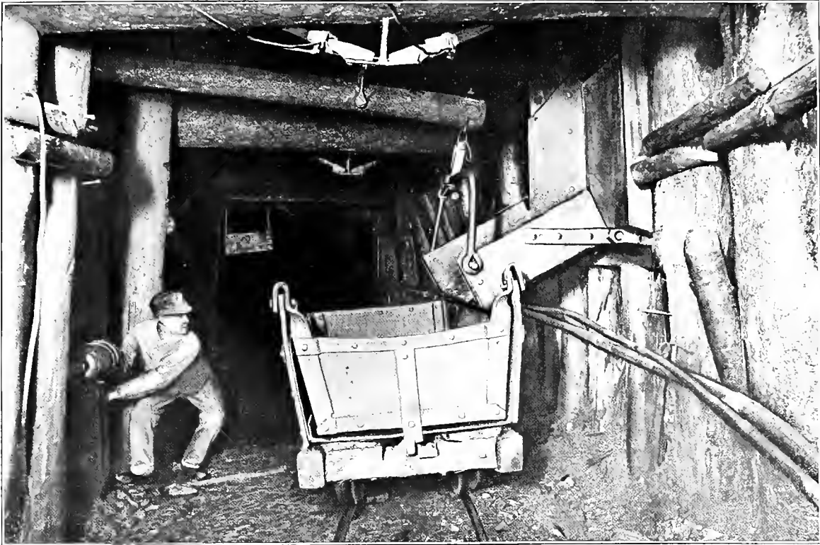
A. VIEW SHOWING METHOD OF LOADING CARS.
