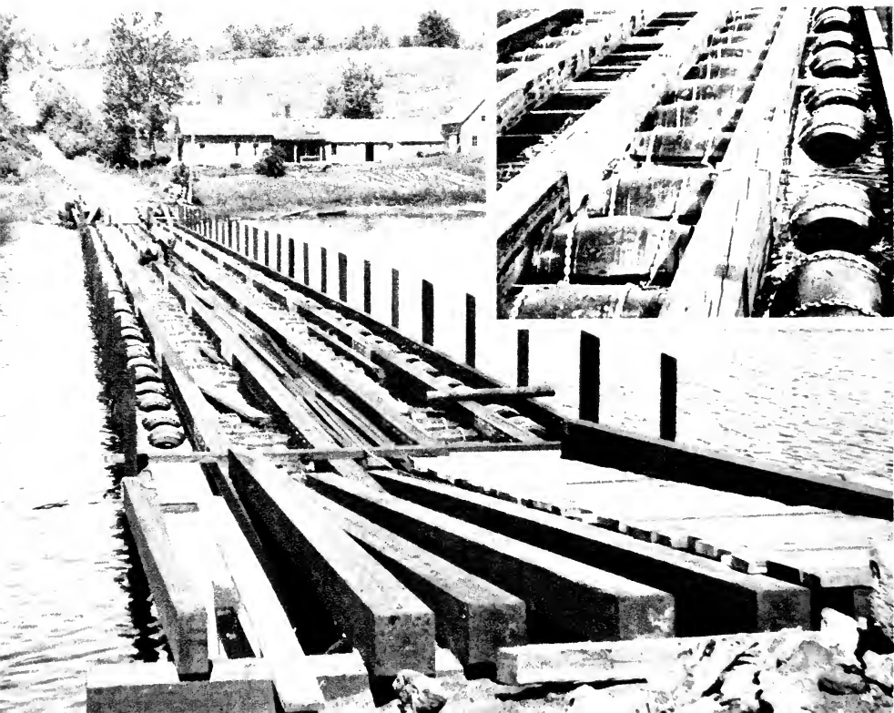
BROOKFIELD FLOATING BRIDGE With inset showing detail of construction
