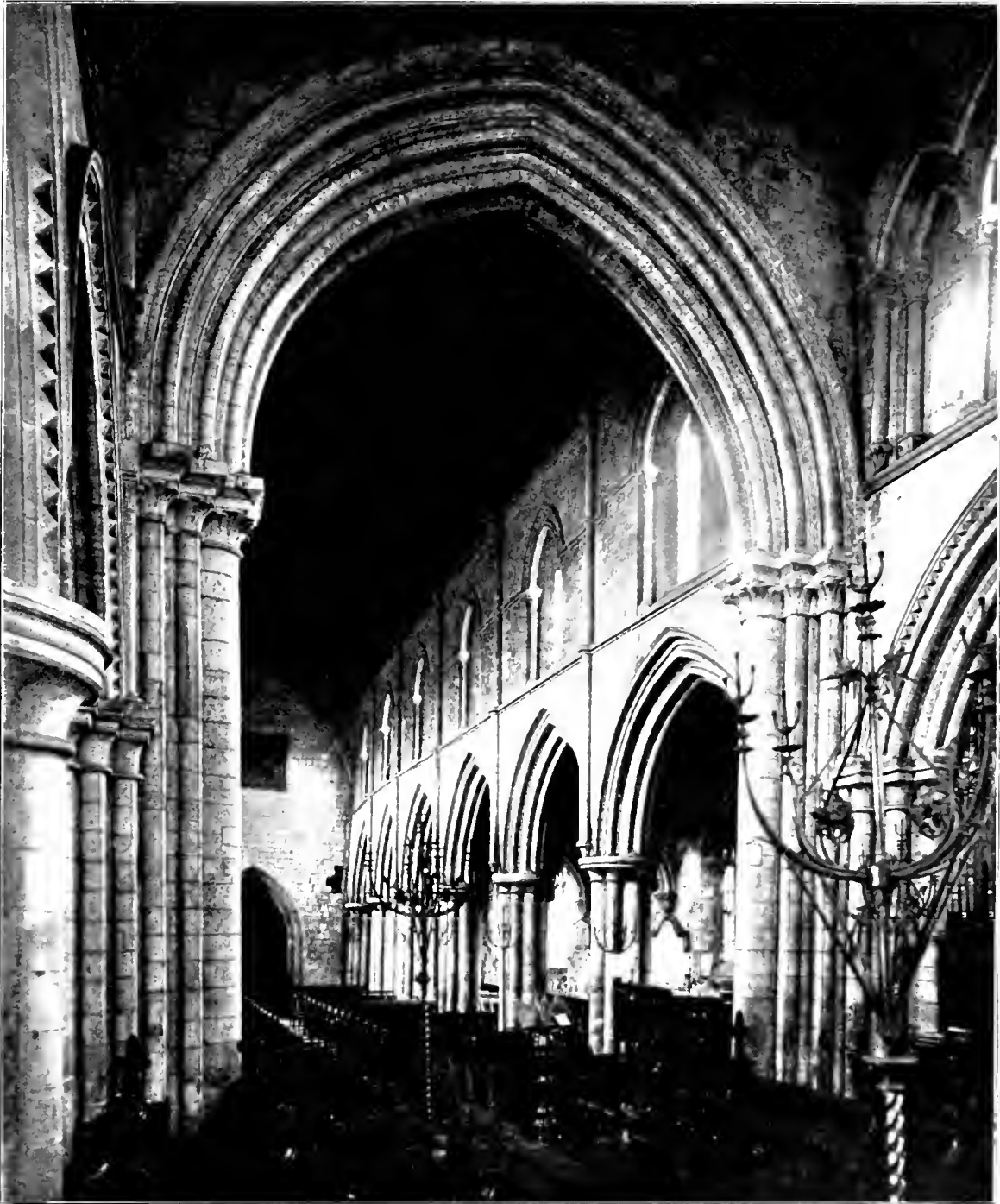
HARTLEPOOL CHURCH: THE CHANCEL ARCH AND NAVE ARCADE
