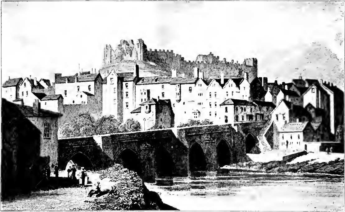
DURHAM: ELVET BRIDGE c. 1829 (By W. Westall)
