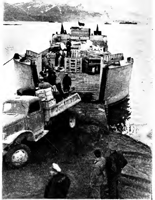
Seabees Unloading Supplies for Base From an LCT Boat at a Point Along the Attu Island Shoreline
