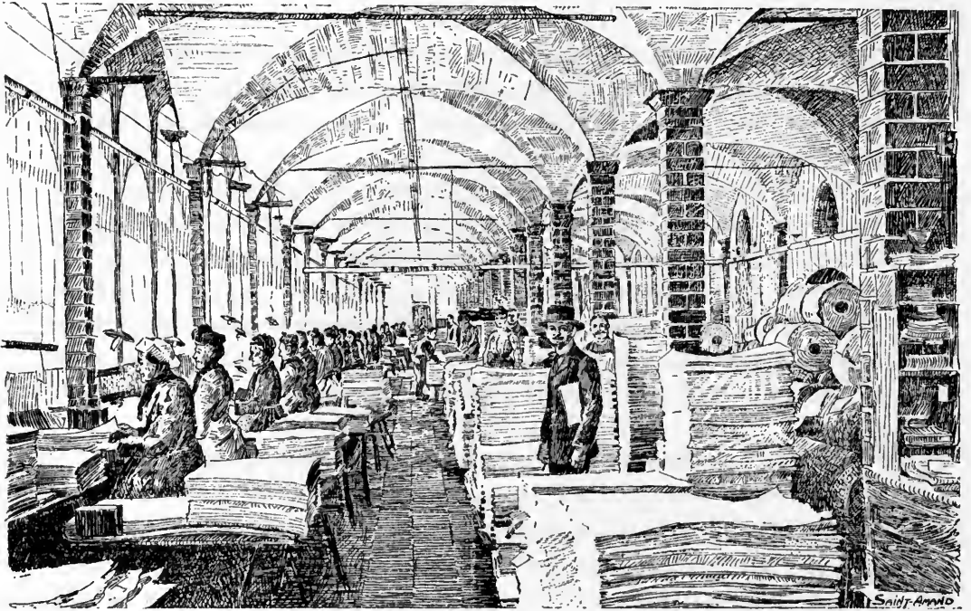
Inspection and selection of sheets
