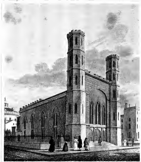
View of the Front
