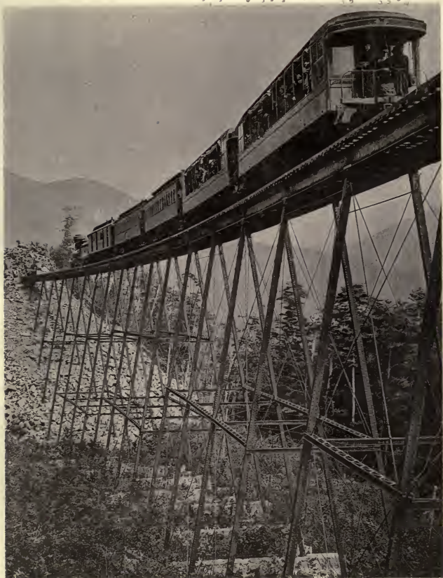
THE FRANKENSTEIN TRESTLE.
