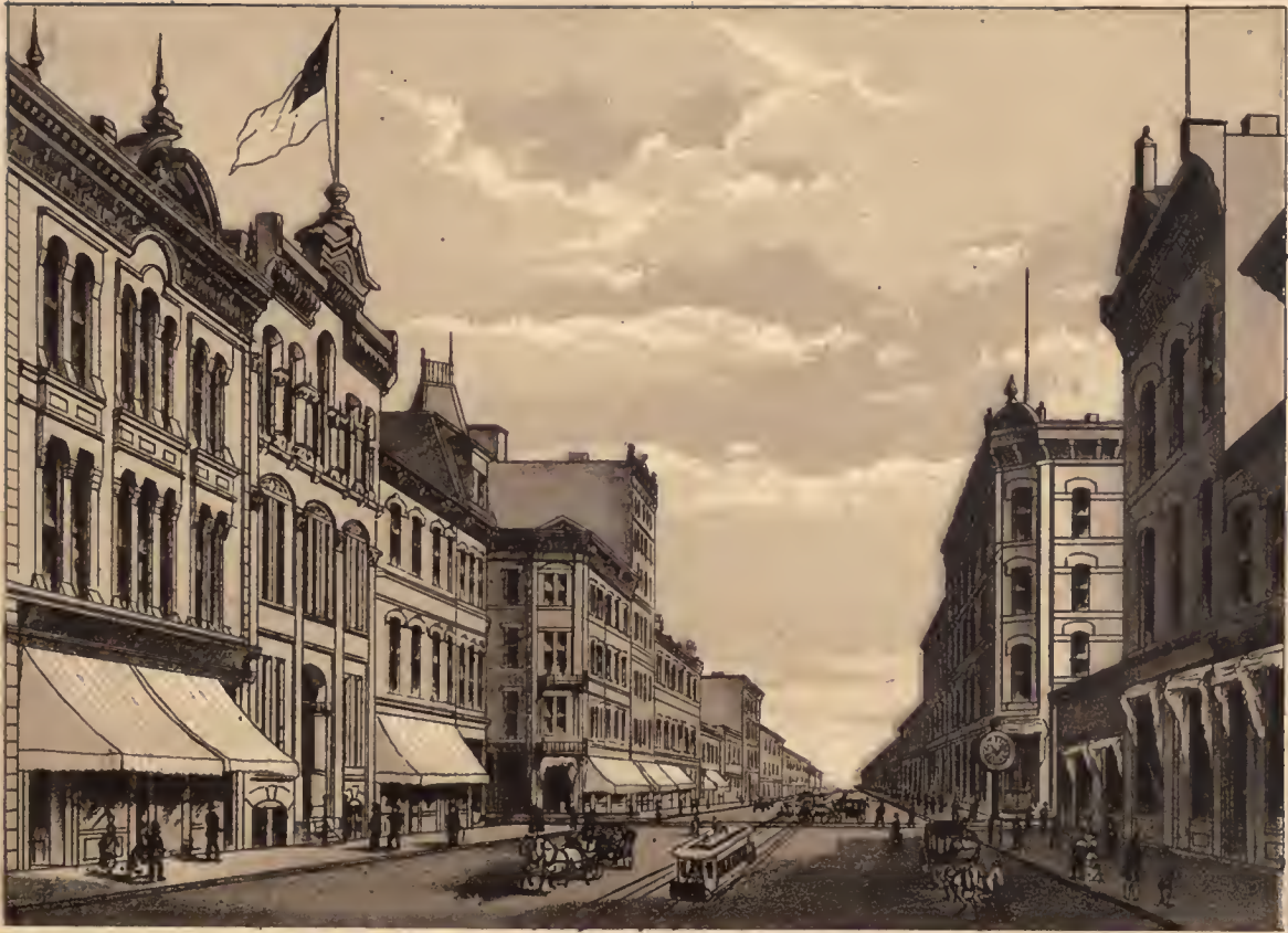
View on Lawrence Street, from Fifteenth Street.
