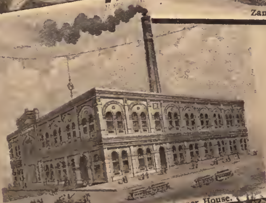
Denver City Cable Co.'s Power House.
