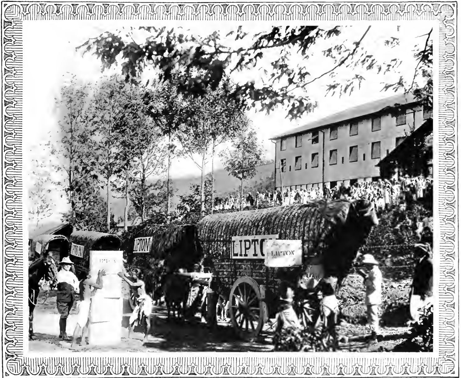
Wagons being loaded at Dambattenne Estate.
