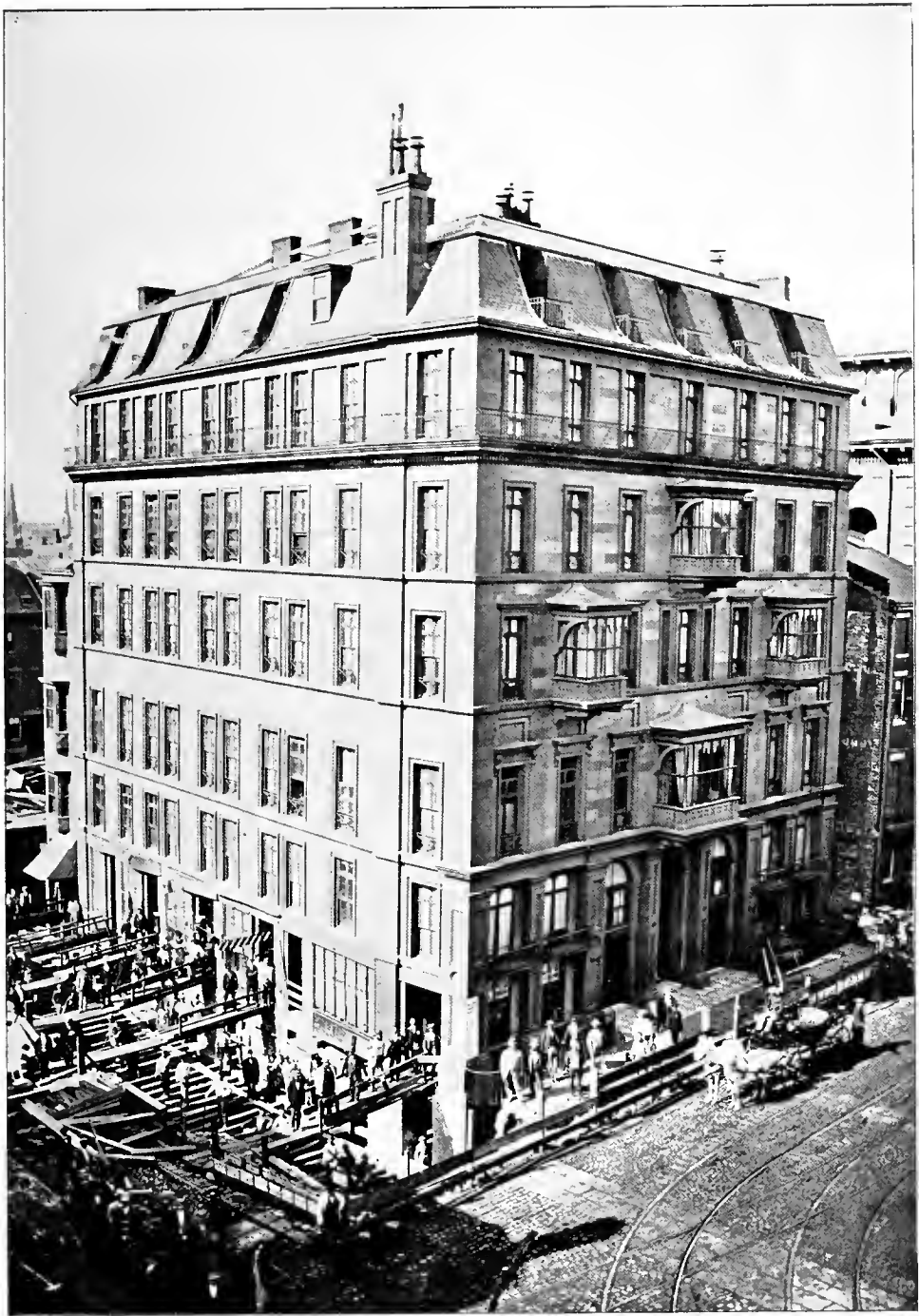
VII.a. — REMOVAL OF HOTEL PELHAM, 1869.
