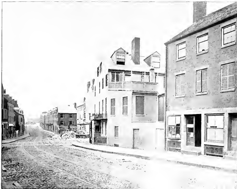
VI.g. — TREMONT STREET BEFORE WIDENING, 1869. Looking South from Warrenton Street.
