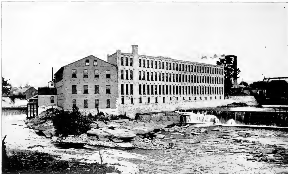
NEW ADDITION TO BAGLEY & SEWALL CO.'S PLANT.
