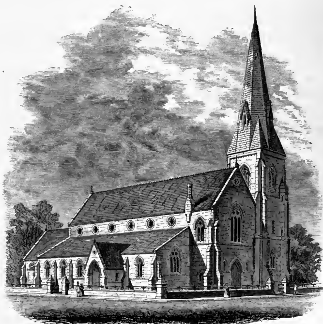
PRESBYTERIAN CHURCH, NEWBURGH. F. C. WITHEES, ARCHITECT.
