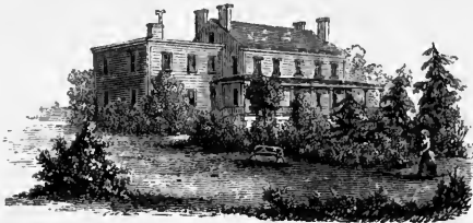
SOUTH-EAST VIEW BEFORE ALTERATION.
