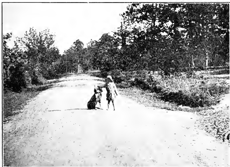
A WELL-KEPT ROAD
