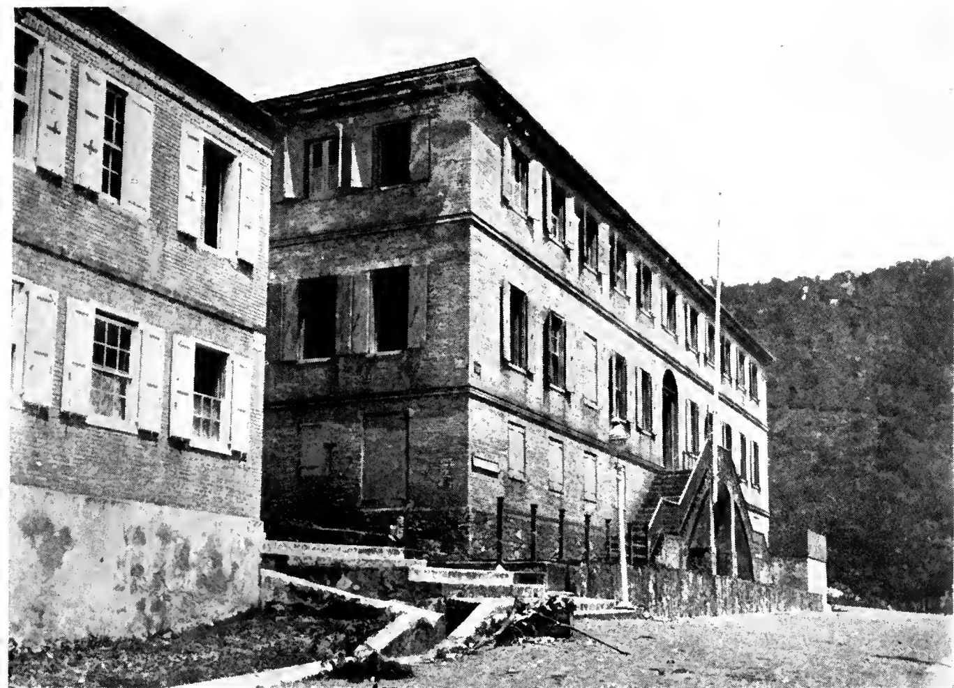
Communal School Building, St. Thomas
