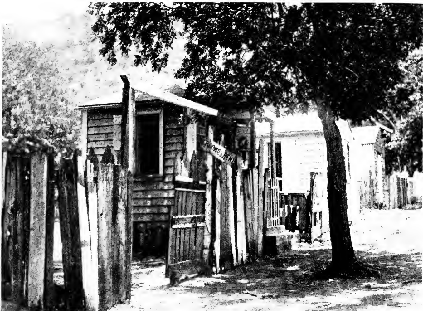
“ Rooms to Rent ”
