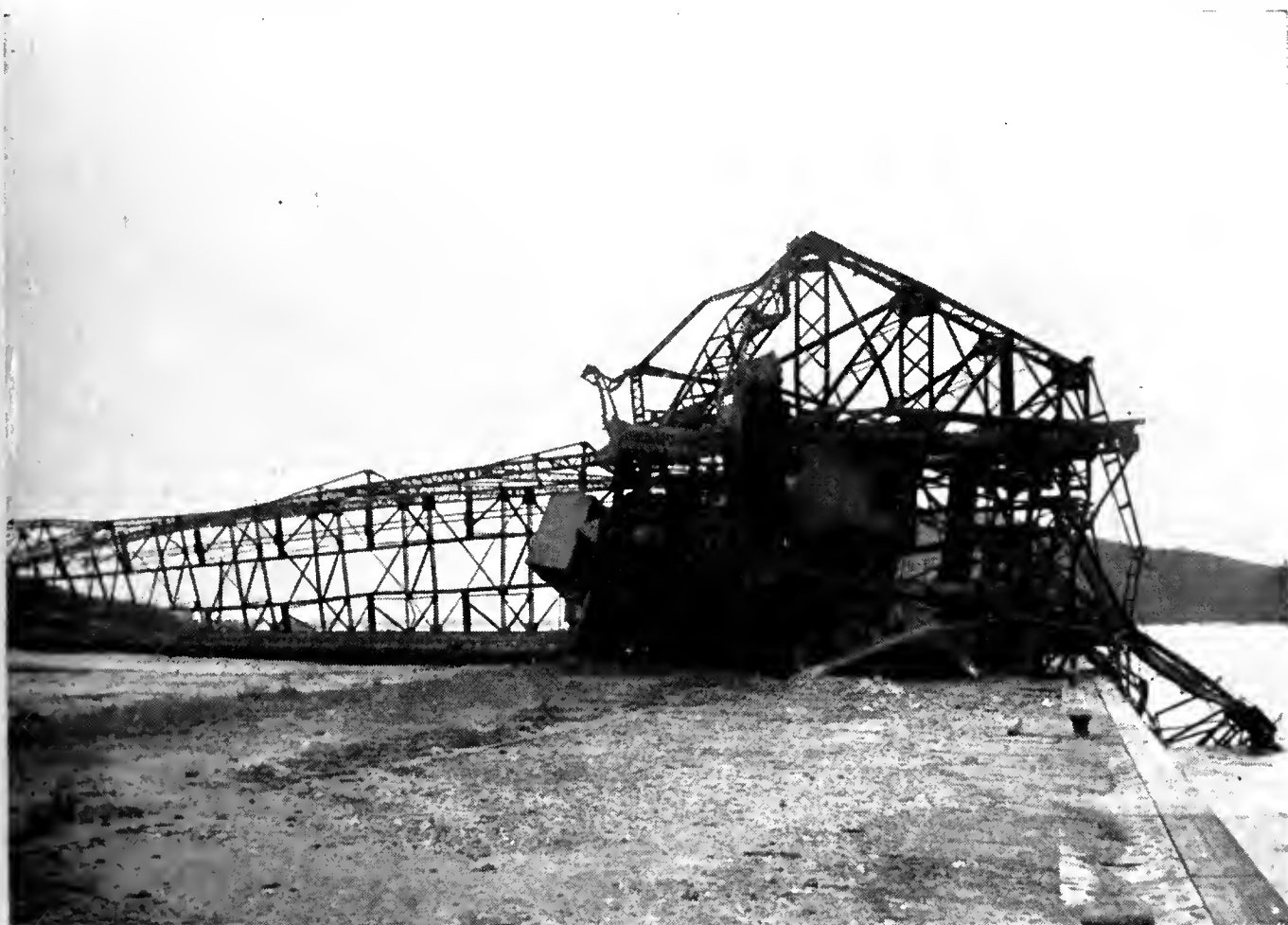
Huge Coal Crane Laid Low by Hurricane
