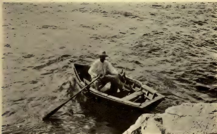
THE ONLY LANDING-PLACE ON CONGO CAY
