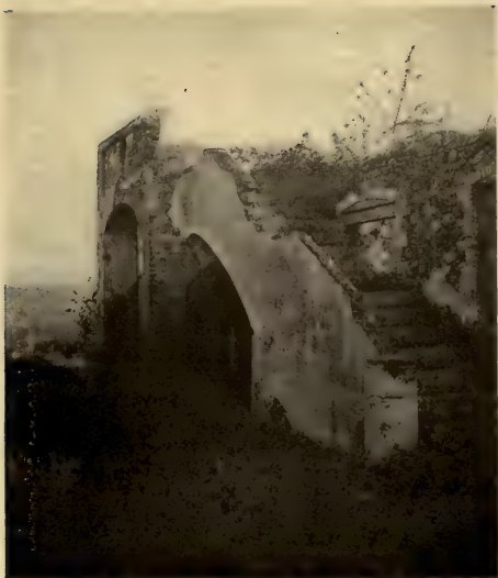
RUINS OF STAIRWAY, NEW HERNHUT MORAVIAN MISSION STATION, ST. THOMAS
