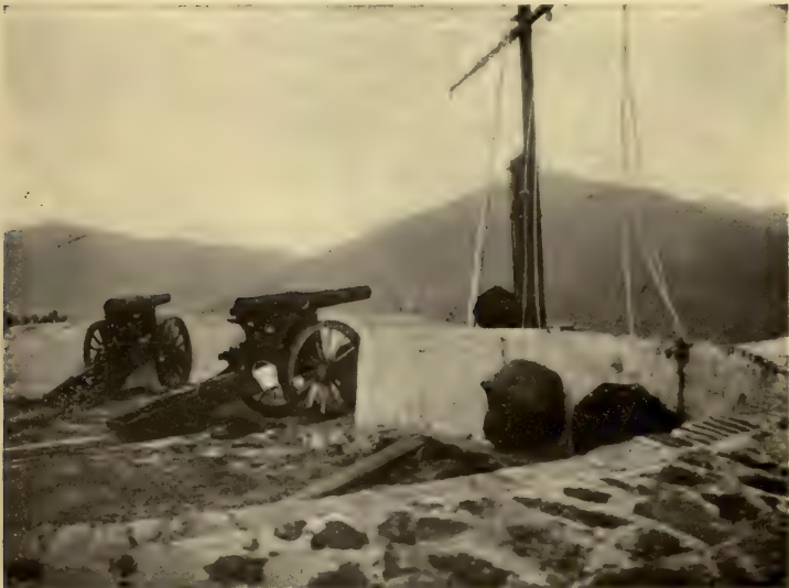
SIGNAL STATION, TOP OF COWELL'S BATTERY
