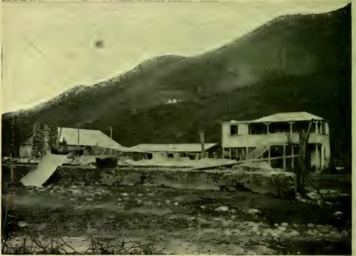
BUILDINGS ON CAROLINE ESTATE, AND BAY-OIL STILL, ST. JOHN
