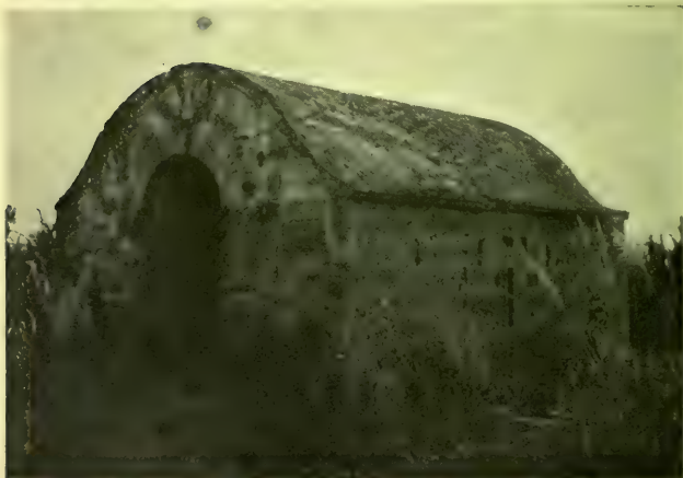
TYPICAL OLD WATCH HOUSE ON SUGAR ESTATE, ST. CROIX
