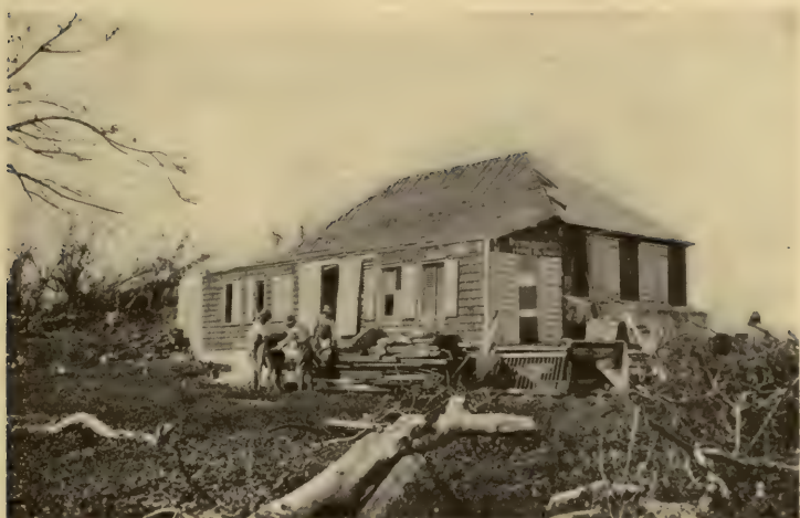
CANAAN ESTATE HOUSE, AFTER HURRICANE
