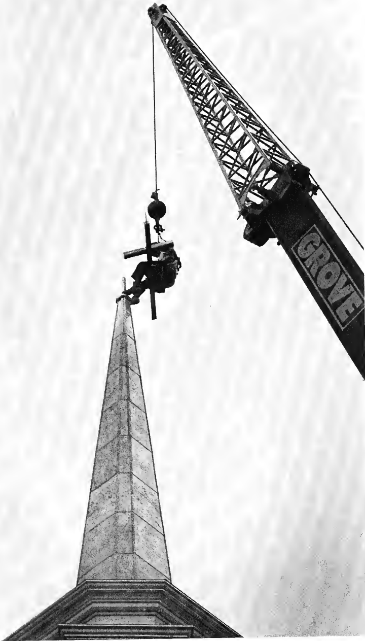
On a very early spring day in 1982, the steeple is put in place, and a cross is hoisted to the pinnacle of the Seby and Christina Jones Chapel.
