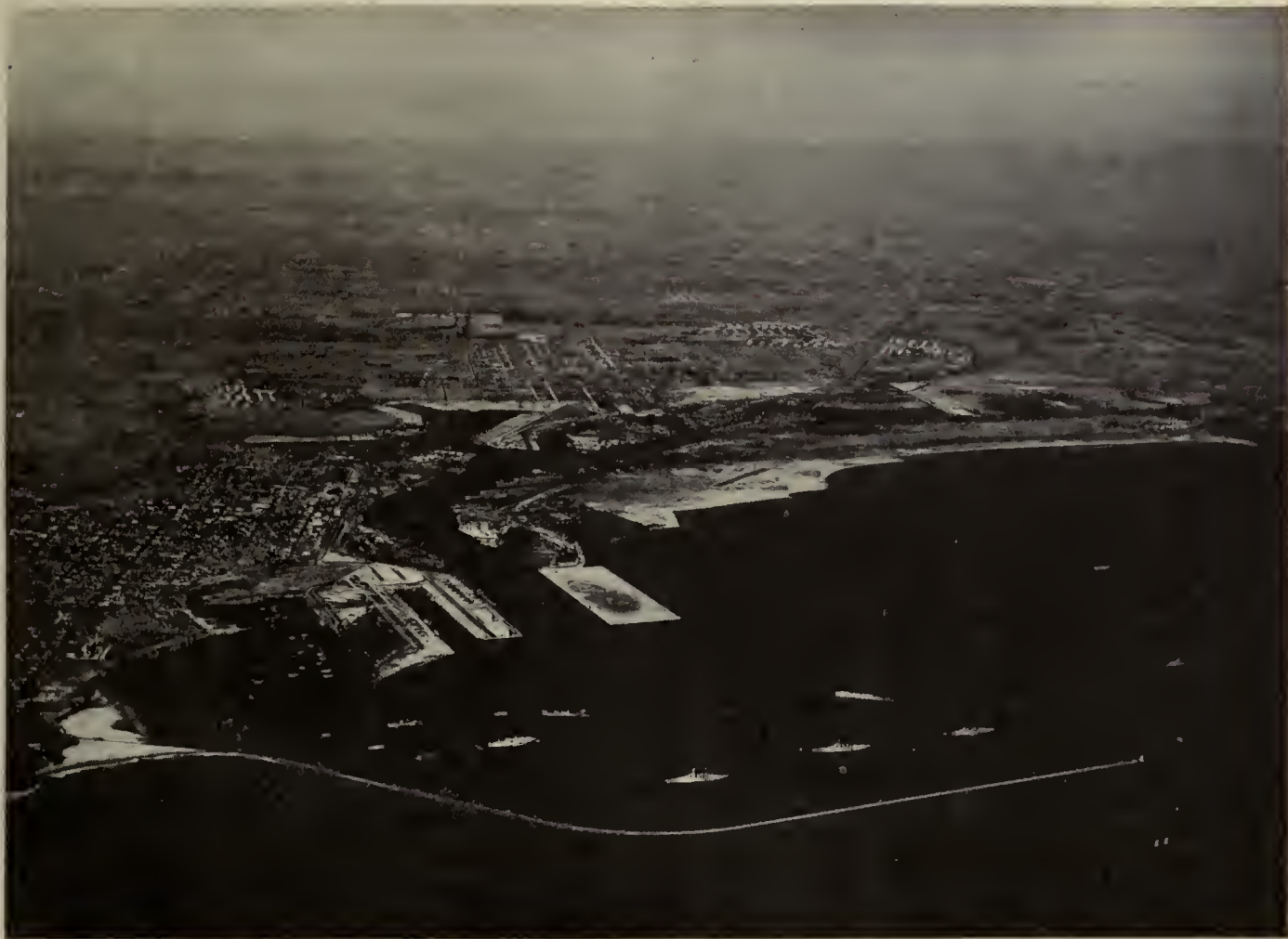
Airview of Los Angeles Harbor—Warships in Foreground
