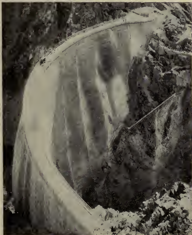
While a Dam Is Being Built the Course of the River is Changed—We See Here How the Finished Dam Looks Before the Water is Turned Back
