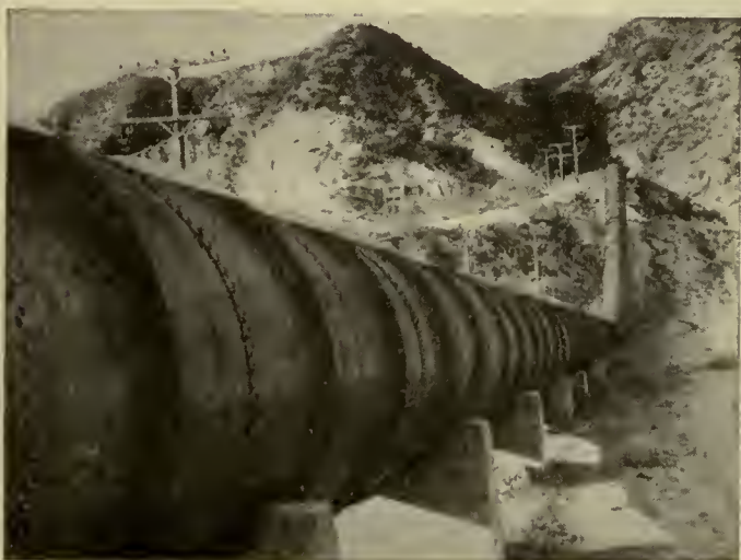
Huge Pipes Carry the Water
