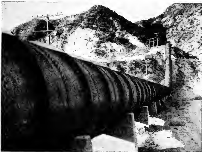
Huge Pipes Carry the Water
